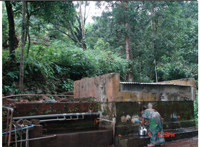
Above: Spring tank with individual water connections. Photo: Parineeta Dandekar
